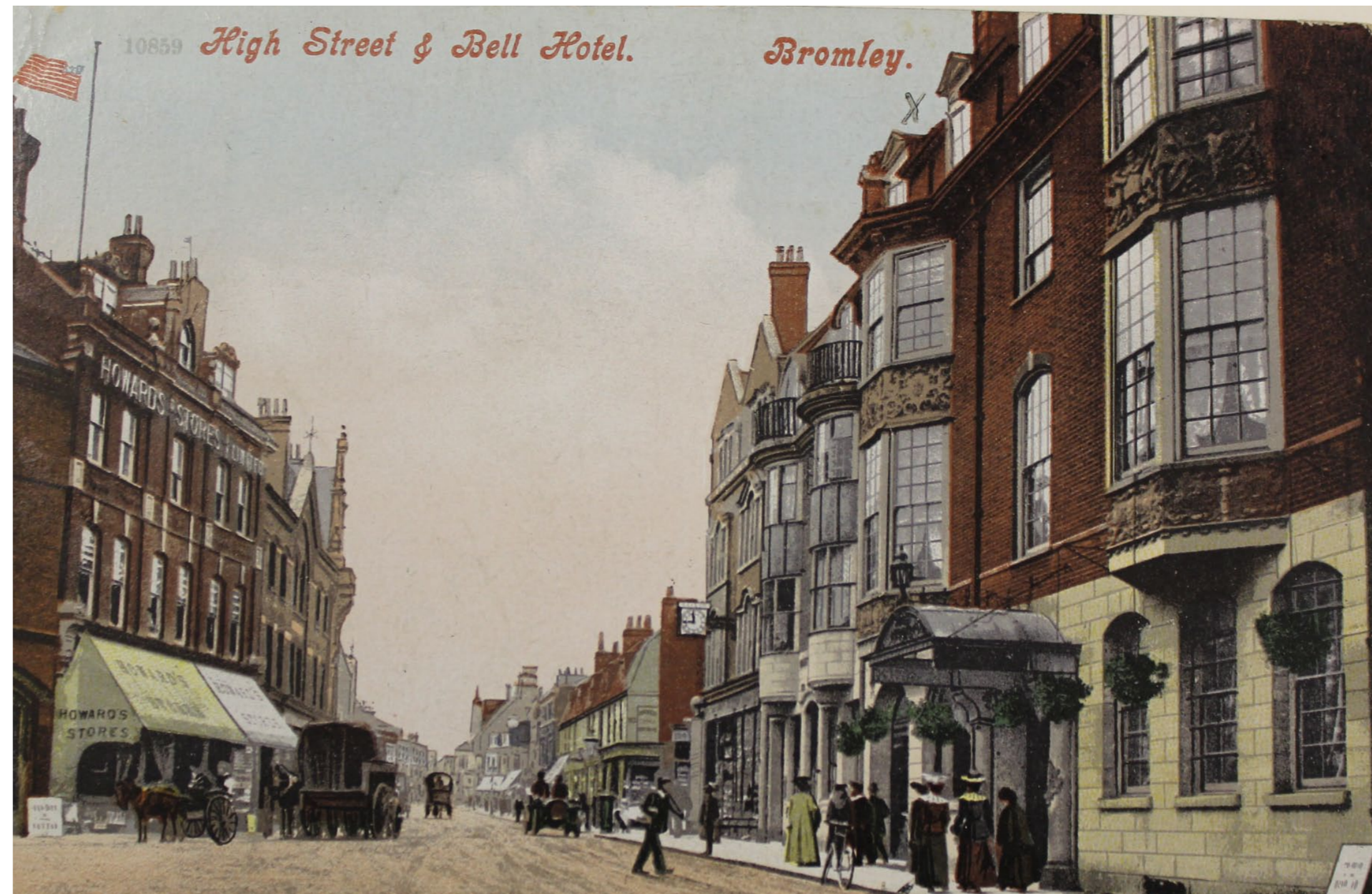
This hand coloured postcard from 1906 shows that the decorative plaster parquetry to the projecting window bays were once painted a terracotta tone. We would like to reinstate this original colour scheme as part of the Royal Bell restoration. Also visible is the ornate cast iron canopy above the main entrance. This is another historic feature that we would like to re-introduce as part of our restoration strategy.
