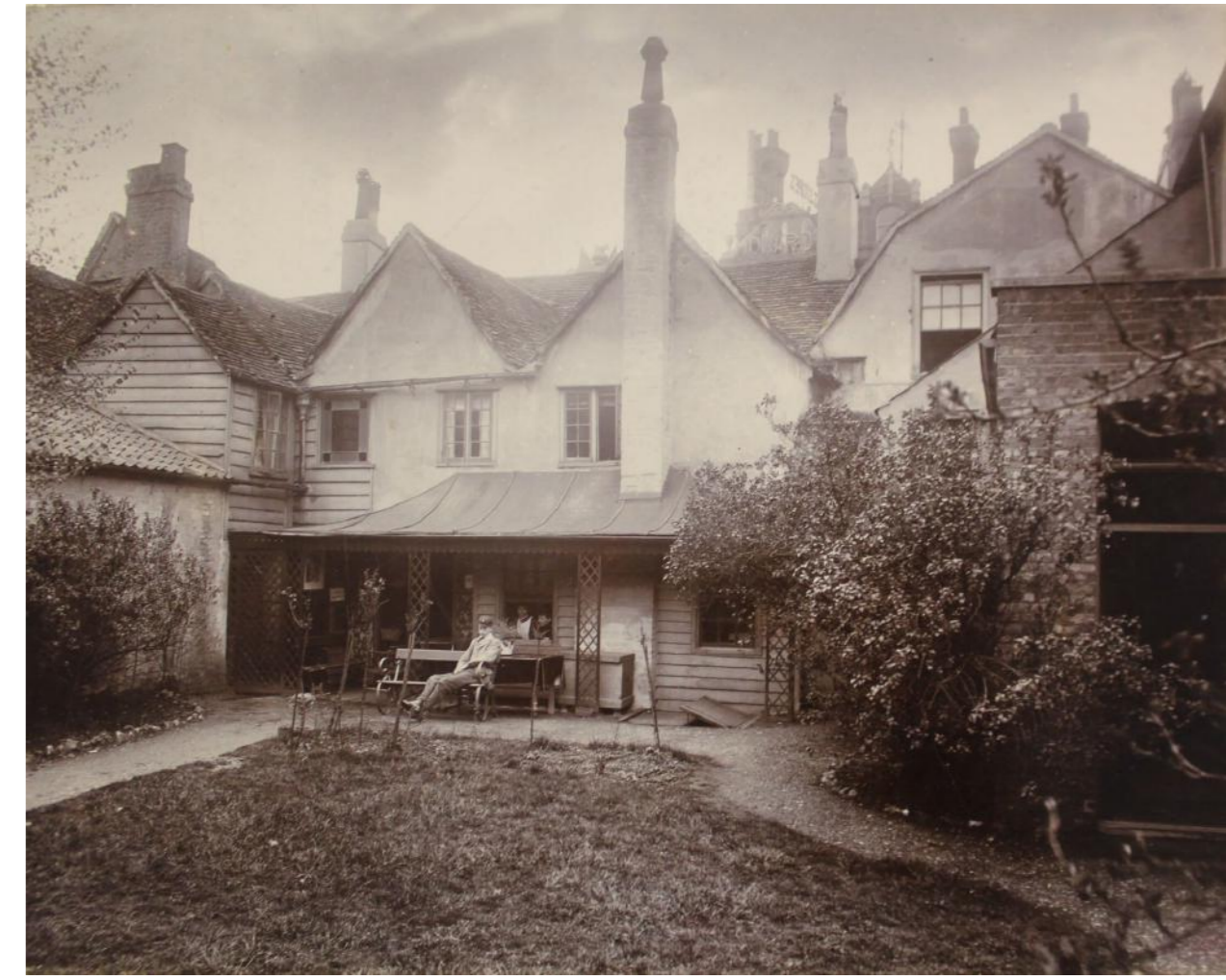
A rear view of the original Royal Bell shortly before its re-building in 1898. It was a timber framed structure with clay tiled roofs.
