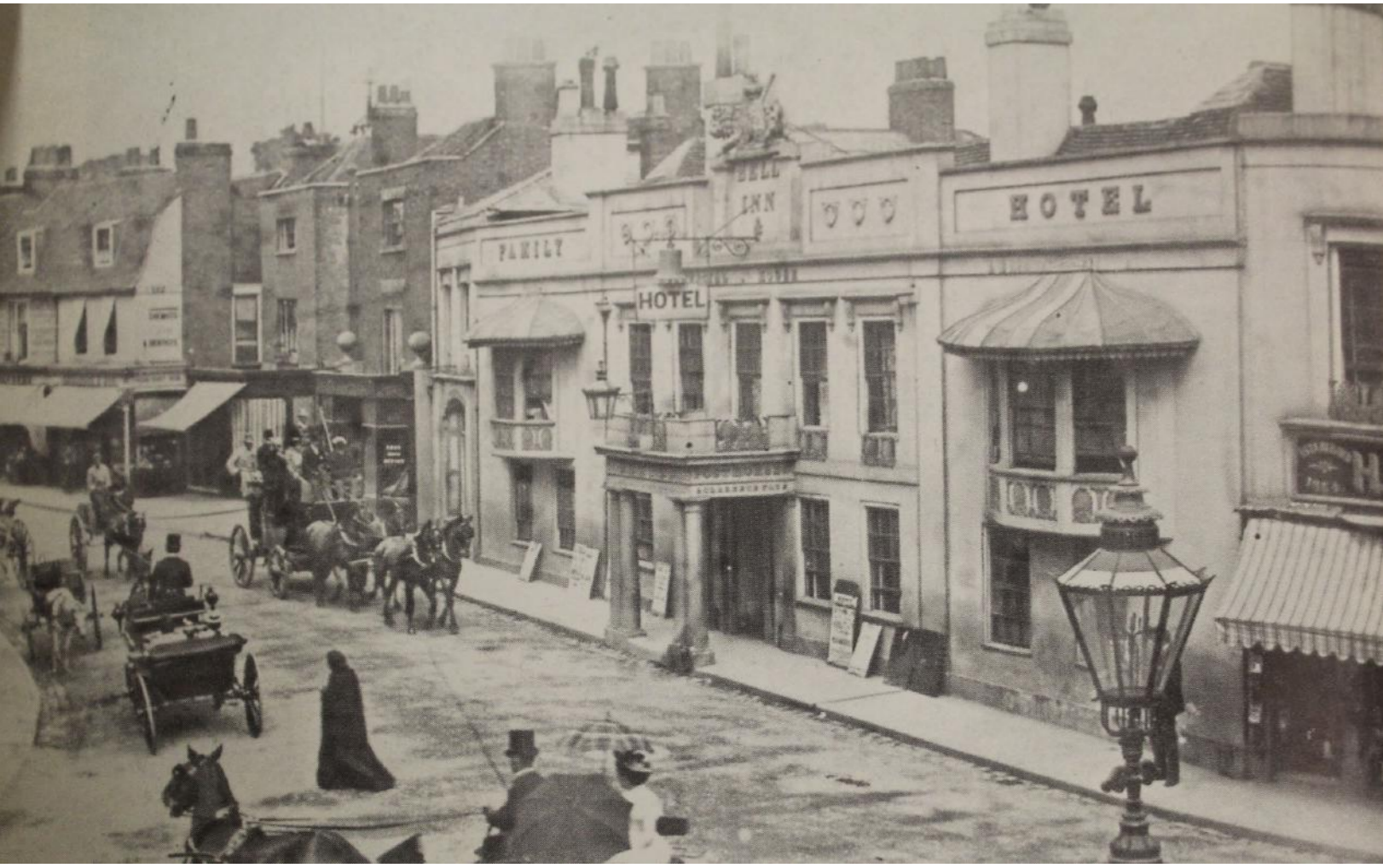
This photograph, circa 1890, shows the original Royal Bell hotel built in the 17th century - one of the important hotels and post houses for Bromley. The stuccoed front and canopied bays are characteristic early 19th century 'Regency' alterations to this venerable landmark for Bromley.
