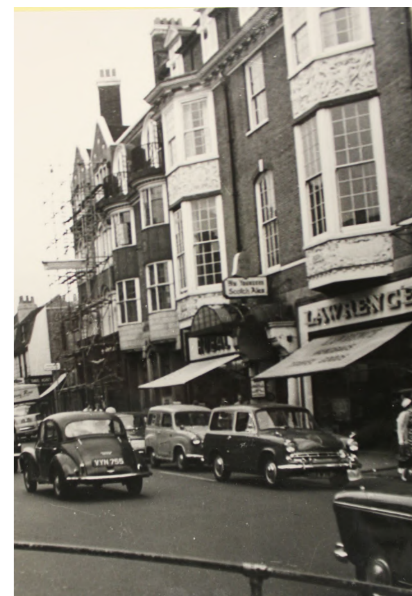
By the mid-20th century new shopfronts had been built into the ground level of the Royal Bell Hotel. We propose to re-introduce traditional shopfronts to these spaces to create an active street frontage to this part of Bromley High Street.
